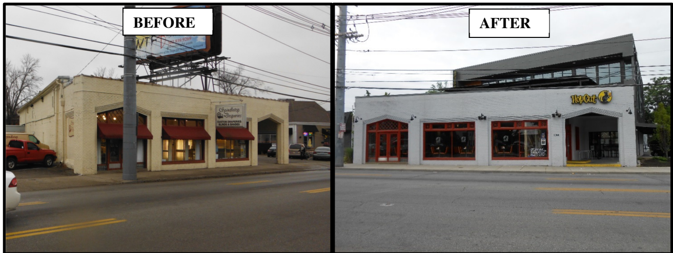
Photo 12: Hopcat restaurant prior to renovation and after completion
