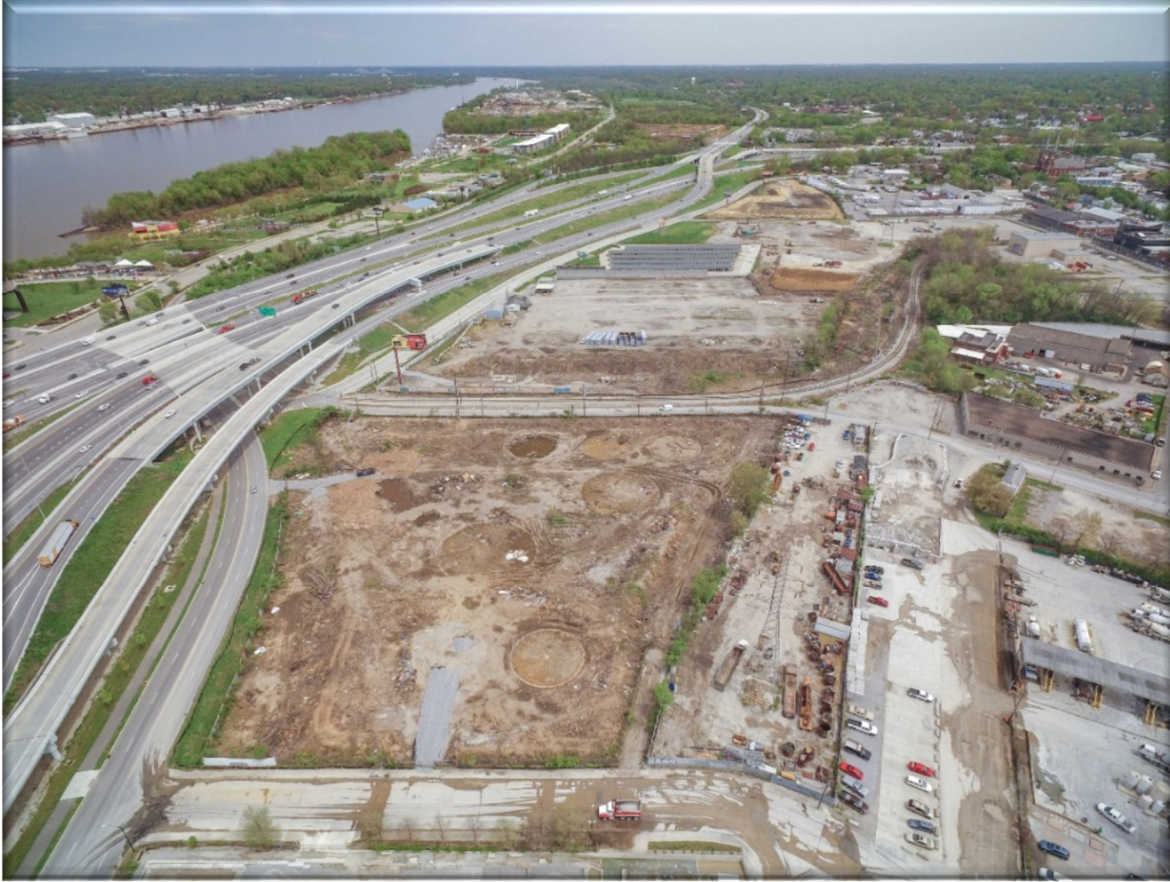
Photo 14: Louisville Soccer Complex, Construction Phase
